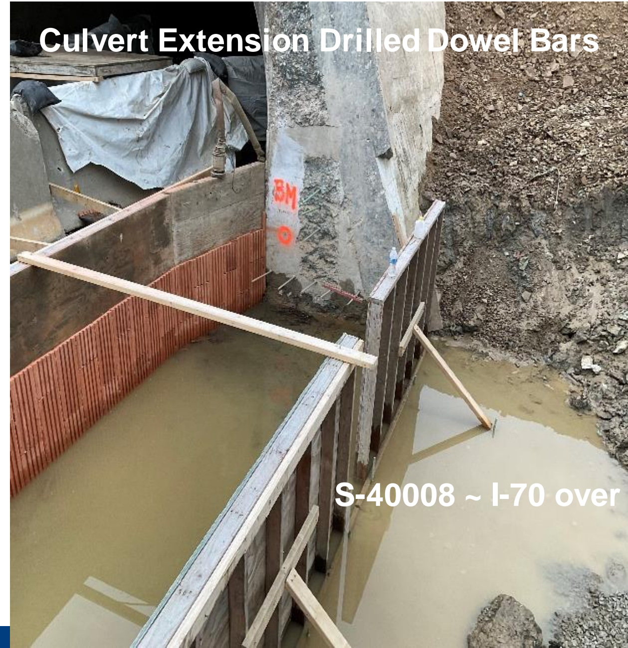
Culvert Extension Rebar Placement
